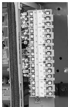
Figure 52. Terminal block on swing plate
