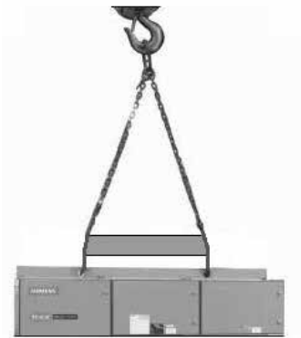
Figure 1. Lifting a motor control center with an overhead crane.
