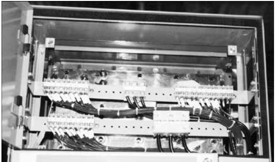
Figure 46. Type "C" wiring terminal
