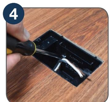
**4** Adjust box height to achieve a flush position; wire the included device and install the gasket and cover
