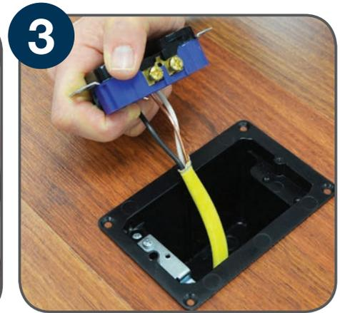
3 Bring the electrical cable through the preferred box clamp, and place the box down in the hole and secure it with the preferred mounting method. Wire the device according to local electrical code.
