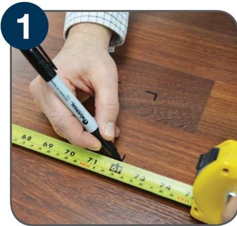
1 Find a location in between floor joists and measure the box dimensions according to the template supplied in the installation instruction sheet.
