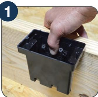
**1** Find and install floor box on solid floor joist; mount with slider plate in the "up" position
