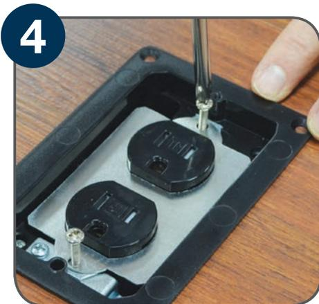
4 Once the device has been wired, secure the device and dust plate down into the box using the screws supplied in the packaging.
